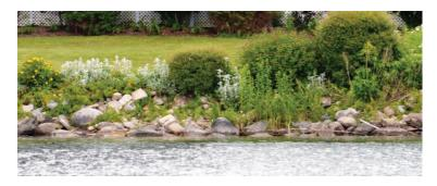
Vegetated Rip-Rap—The stones prevent erosion along the shoreline from wave action while the vegetation roots into the soil, binding it into place.
